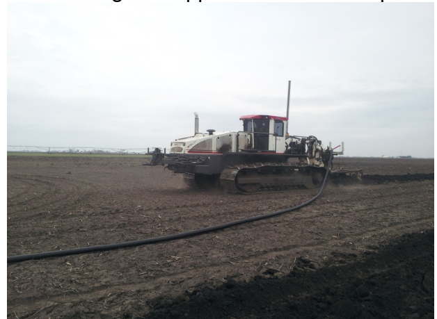
Corrugated HDPE pipe is installed at the Monsanto research farm.
